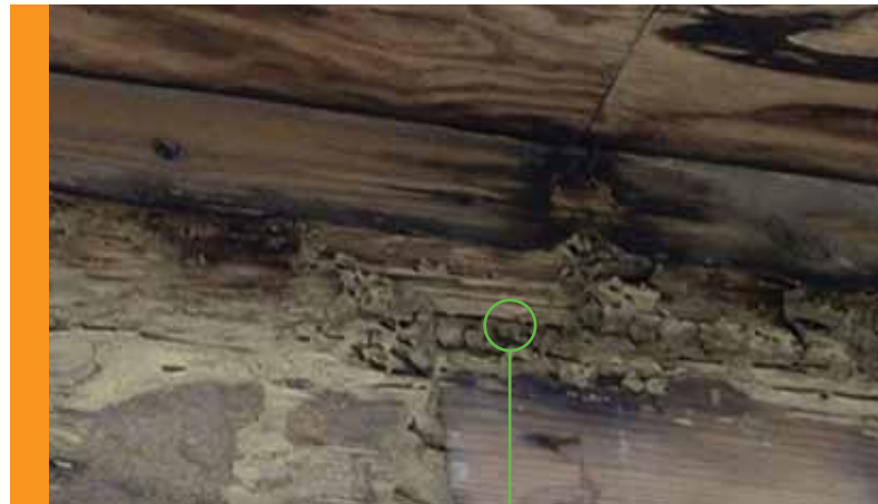
● Termite Damage
